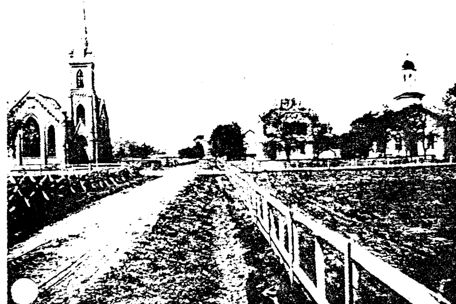
Brick church built in 1892-93 Frame parsonage built in 1879
